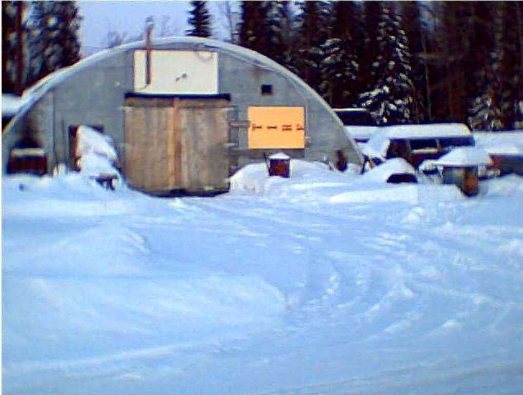
Existing industrial use – industrial shed
