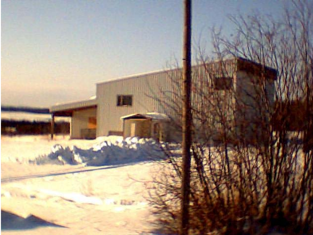
Existing industrial building
