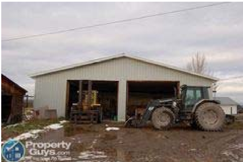
Existing Industrial – 1,800 sq ft heated shop
